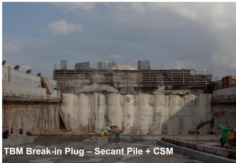
Figure 4. Port Miami Tunnel (POMT) TBM Break-in Support of Excavation With Secant Pile And Cutter Soil Mixing Wall
