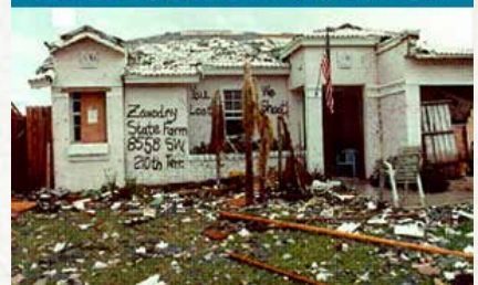
Level 3 - Major damage; uninhabitable
