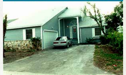
Level 2 - Major damage; habitable
