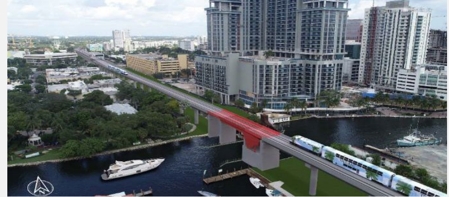
56-foot mid-level bascule
