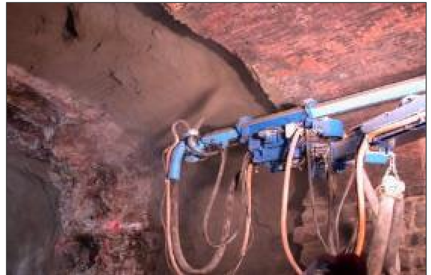
Figure 30: Construction During SEM Example 2
