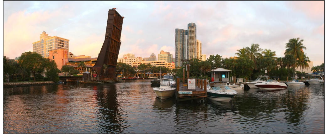
Figure 1: Bascule bridge on New River
