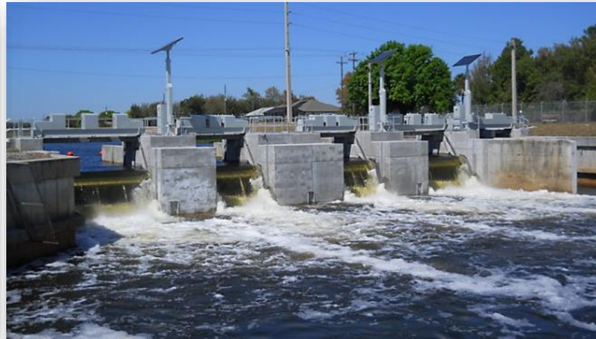
Gravity driven discharge
