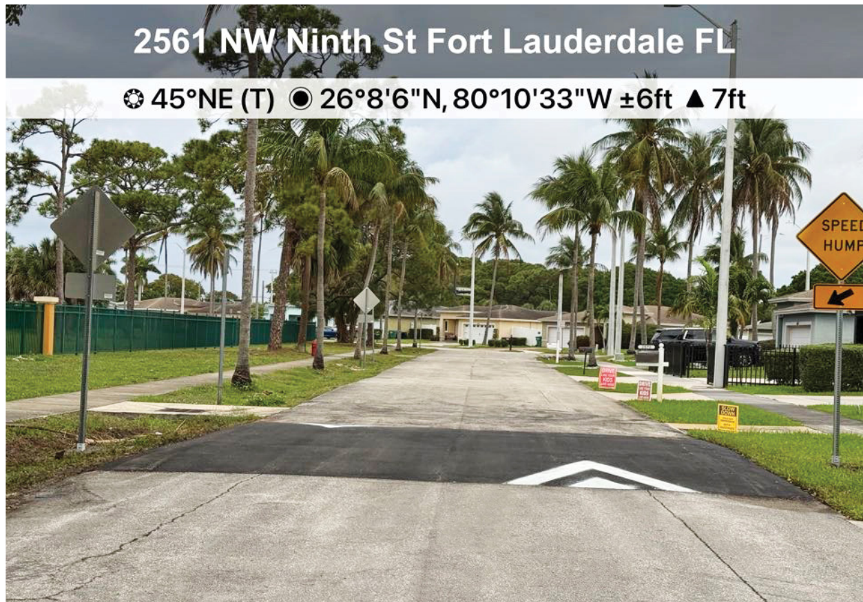
Newly installed speed hump on NW 9th Street
